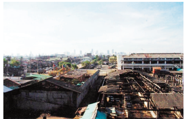
View from the office: Old and dilapidated cow slaughterhouse
